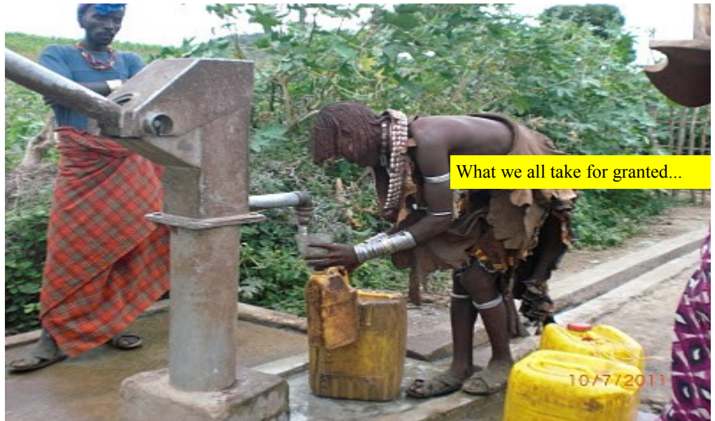
Galcide Water Well The new Galcide well in use!
